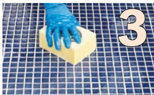
3 Wash any residue off the face of the tiles when slightly hardened in the joints, and up to 60 minutes after application
