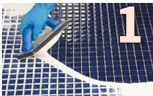
1 Apply ARDEX EG 8 PLUS with a standard squeegee
