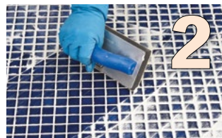
2 Remove excess ARDEX EG 8 PLUS from the surface
