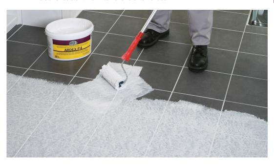
The consistency of ARDEX P 4 Primer virtually eliminates drips and splashes, making it ideal for use on walls, ceilings and floors, on a wide range of absorbent and non-absorbent substrates.
