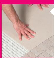
Tiles can then be fixed using any ARDEX Cement-Based Tile Adhesive, approximately 60 minutes after the application of the second coat of MIX TWO.
