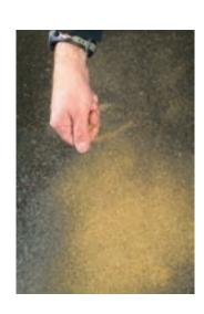
**ARDEX Aggregates** are perfect for fully blinding epoxy primers.
