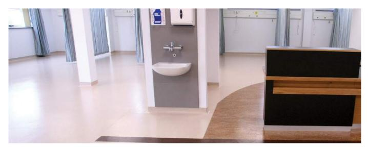
If preferred, the floorcovering or profile can be pre-coated the day before installation. The open time for flooring/profiles already pre-coated on the previous day into the newly applied film is approximately 90 minutes. The surfaces coated/pre-coated with ARDEX AF 620 must be placed together within the open time of 24 hours.
