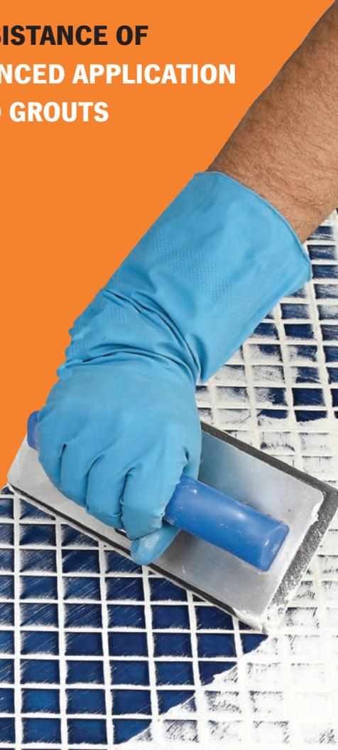
**ARDEX EG 8 PLUS** is an epoxy tile grout and adhesive with excellent resistance to most chemicals but, unlike traditional epoxies, it is easy to apply, requires no special tools and can be cleaned off the tile surface in as little as 15 minutes and up to 60 minutes after application.
