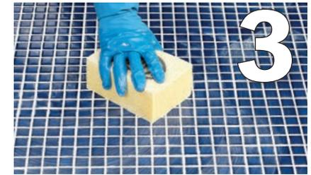
Wash off any residue when the grout is slightly hardened in the joints, in as little as 15 minutes and up to 60 minutes after application
