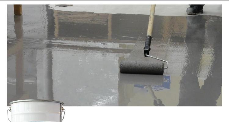
**ARDEX WPM 200** has been specifically developed to provide a water and water vapour barrier to concrete, screeded, rendered or masonry surfaces, steel and other hard surfaces.
