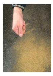
**ARDEX Aggregates** are for use with ARDEX Subfloor Smoothing compounds where thicker applications are required, or for fully blinding epoxy primers.
