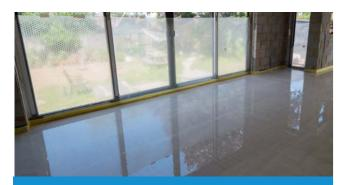
Ensure appropriate site climatic conditions, for example, a reasonable indoor temperature and relative humidity, and through heating and ventilation in accordance with BS EN 13813.
