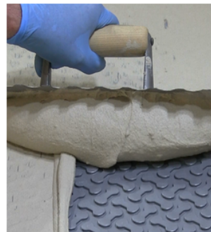
Tile immediately with an appropriate ARDEX tile adhesive
