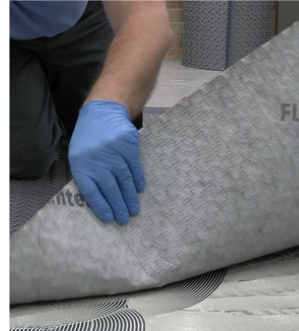
Air for 5 minutes then lay the mat down
