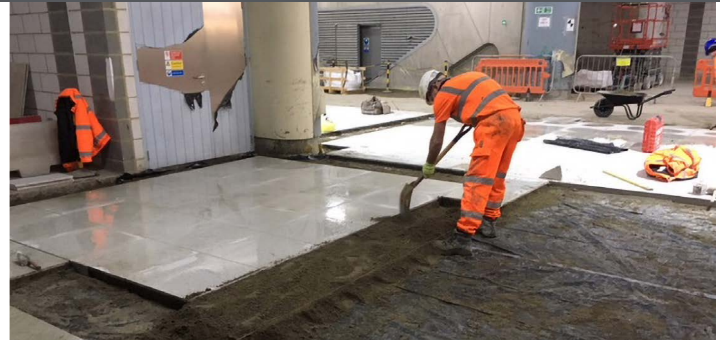
ARDEX A 38 has been used extensively on the London Underground and on projects where fast turnaround is essential.
